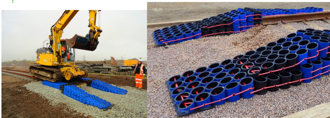
Figure 13 Example of ramp for entry/exit to worksite
