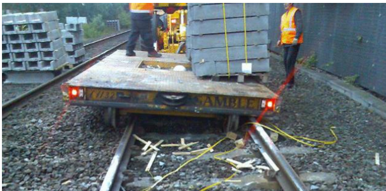
Figure 8 Results of poor unloading sequence (Historical photograph)
