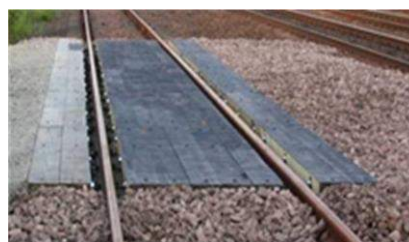
Figure 10 Secured Timbers
