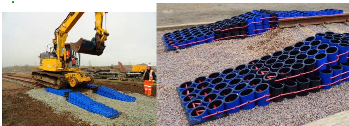
Figure 13 Example of ramp for entry/exit to worksite
