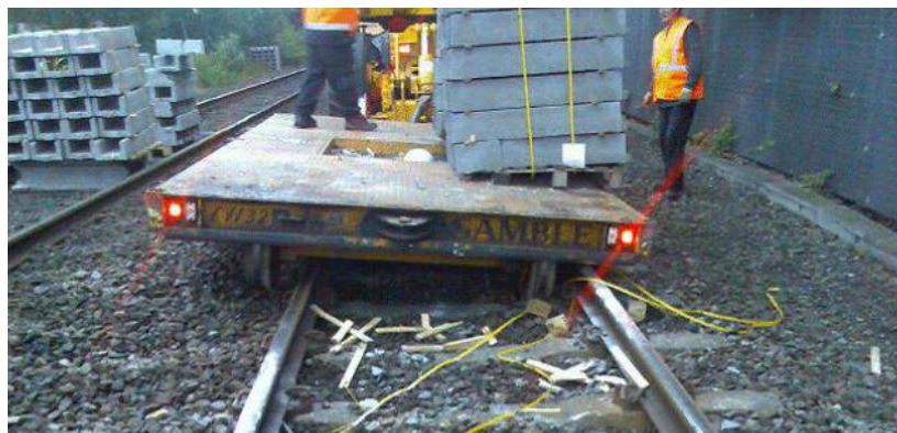
Figure 4 Results of poor unloading sequence (Historical photograph)
